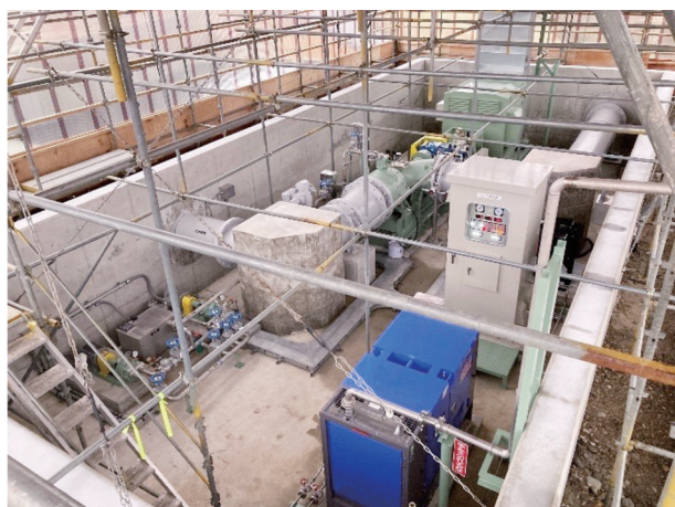
図11 現地据付状況 Fig.11 On-site installation status
