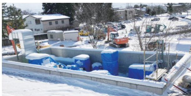
図9 現地施工状況 Fig.9 On-site construction status
