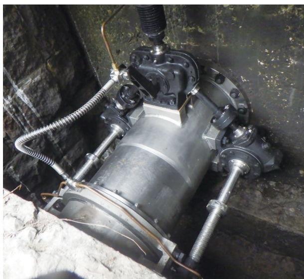
図6 導水弁2号の更新状況 Fig.6 Post-Renewal Condition of HBV No.2
