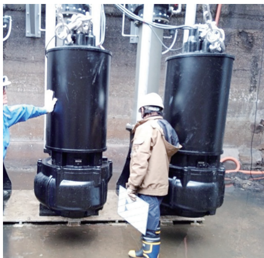
図6 仮設ポンプ外観 Fig.6 View of temporary pump
