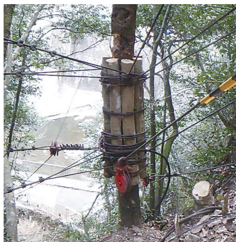
図3 木に固定 Fig.3 Secure the wire to the tree
