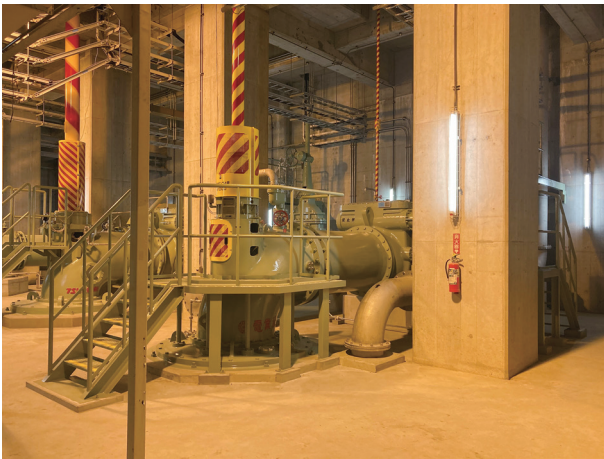
図7 現地据付後の污水ポンプ4号 Fig.7 View of the No.4 pump at site
