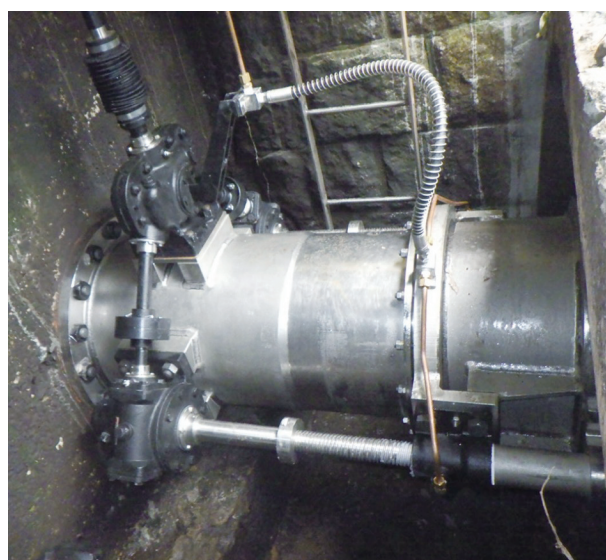
図7 導水弁1号の更新状況 Fig.7 Post-Renewal Condition of HBV No.1
