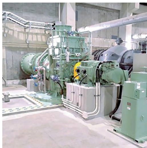
図3 No.1雨水ポンプ外観 Fig. 3 View of No.1 rainwater pump
