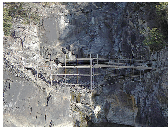
図5 岸壁の仮設足場 Fig.5 Temporary scaffolding on the rock fac
