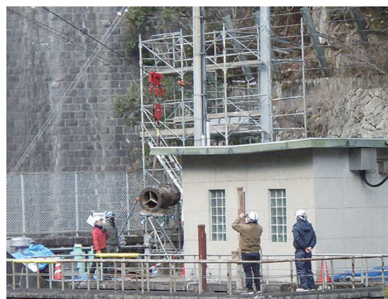
図4 仮設に固定 Fig.4 Secure the wire to the Temporary scaffolding
