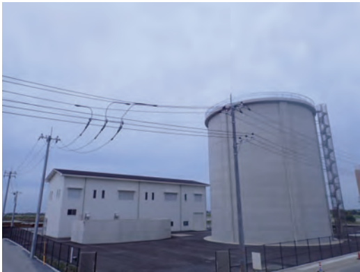
図2 機場全景 Fig.2 View of pumping station
