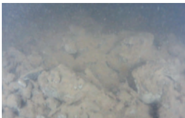
図4 排水機場水槽内 Fig.4 Pump station sump
