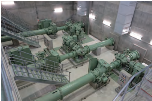
図6 用水ポンプ据付完成状況 Fig.6 View of the pumps after installation
