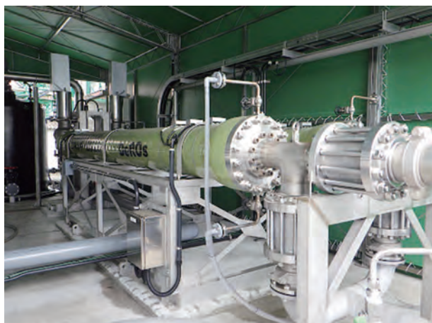
図4 ERD外観 Fig.4 View of ERD
