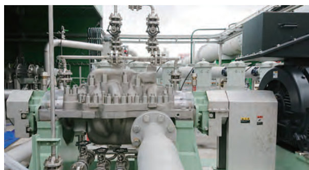
図7 高圧ポンプ外観 Fig.7 View of high-pressure pump
