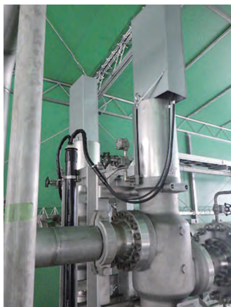
図5 切替弁外観 Fig.5 View of switching valve
